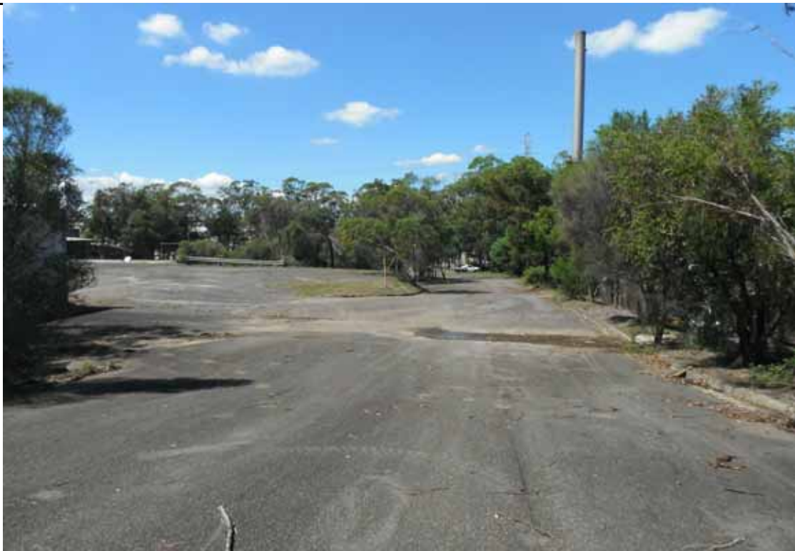
Photograph 3 - Internal road on west of property
